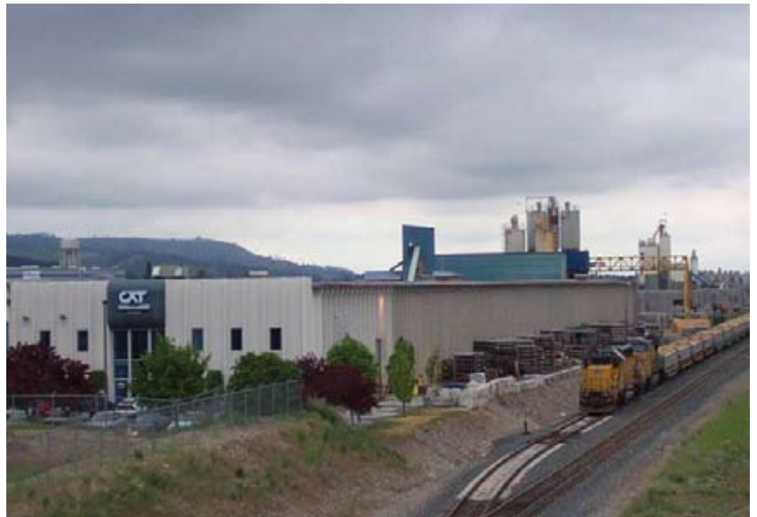
Spokane, Washington Facility
