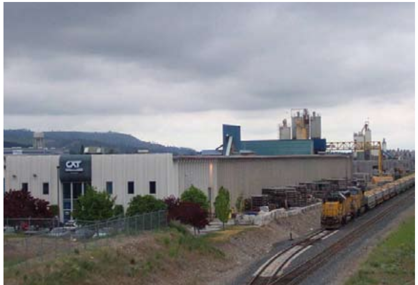
Spokane, Washington Facility
