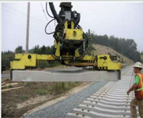
Efficient installation using hydraulic clamp
