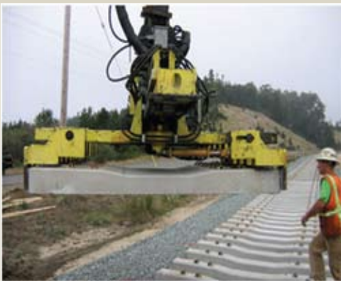
Efficient installation using hydraulic clamp
