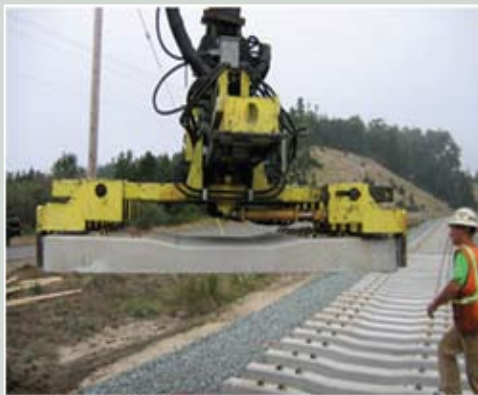
Efficient installation using hydraulic clamp
