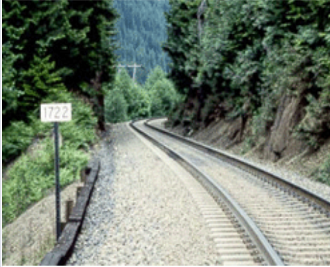
Concrete ties with Safelok fastening system
