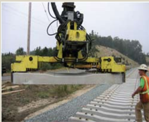
Efficient installation using hydraulic clamp
